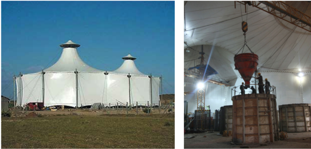
Precast concrete mobile factory in Gujarat, India
